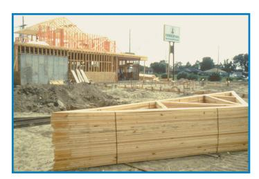
Plan ahead! A semi trailer truck delivers your trusses. On delivery day, MAKE SURE YOU HAVE PLENTY OF ROOM for the truck to get in and room set aside for the trusses.
