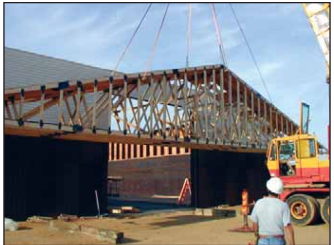
Pick up the finished assembly and set it into place.
