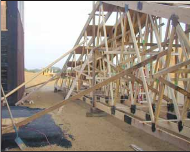
Ground Bracing for truss assembly being built on the ground.
