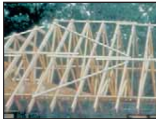
Above: Proper bracing scheme - Continuous TCTLR with Diagonal Bracing. PHOTO B2-7
