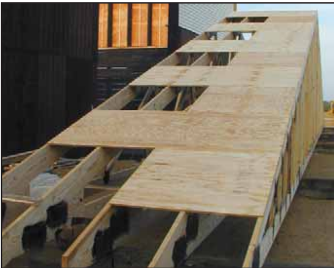
Install Structural Sheathing as soon as the first "set" of trusses have been properly plumbed, restrained and braced.
